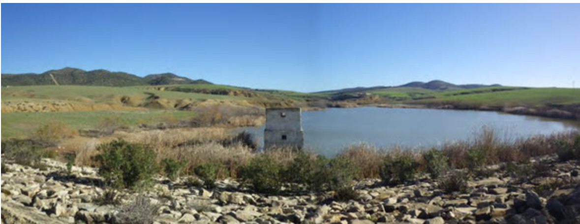
General view of reservoir, BE-2 Labiadh
