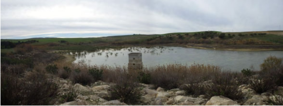
General view of reservoir, SI-5 Erroumi
