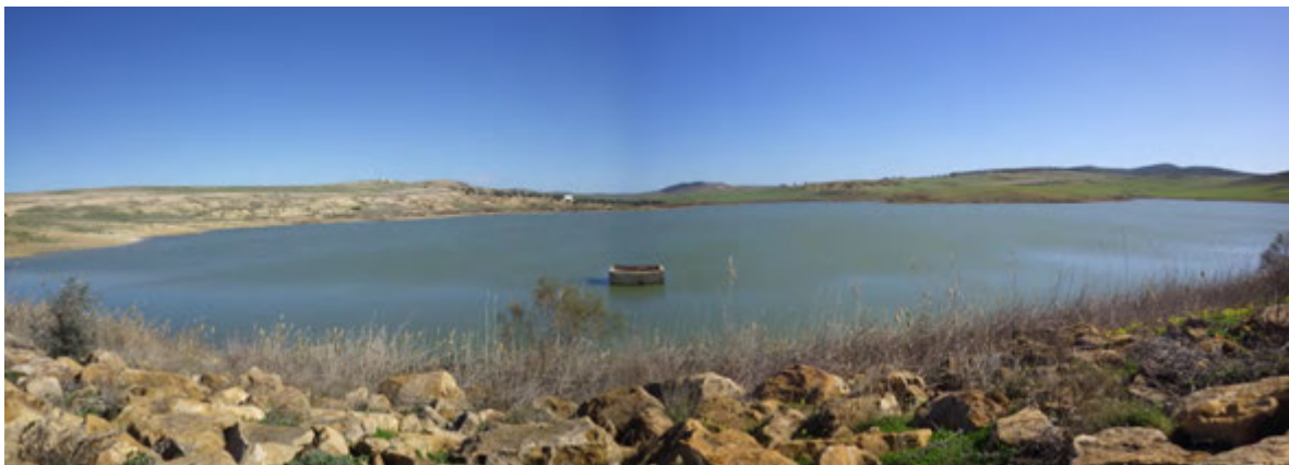
General view of reservoir, BE-5 Sidi Yahia
