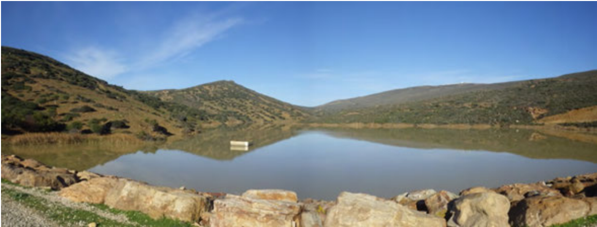
General view of reservoir, NA-1 Tabouda
