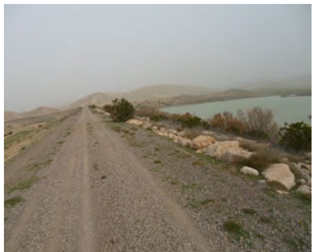
Dam crest and reservoir, KE-2 Rouijel
