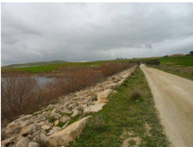
Dam crest and reservoir, KE-1 Bou Yagoum
