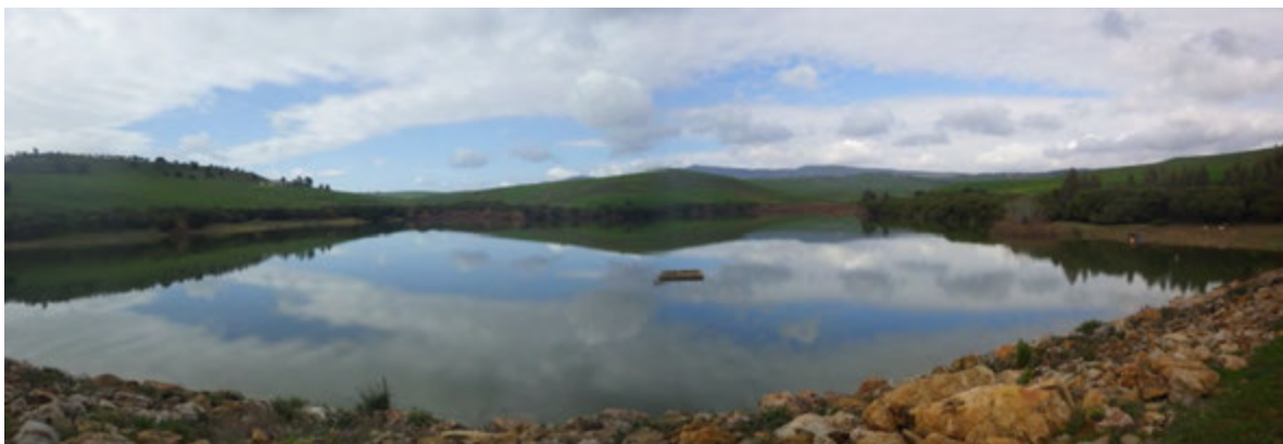
General view of reservoir, JE-1 Sammar
